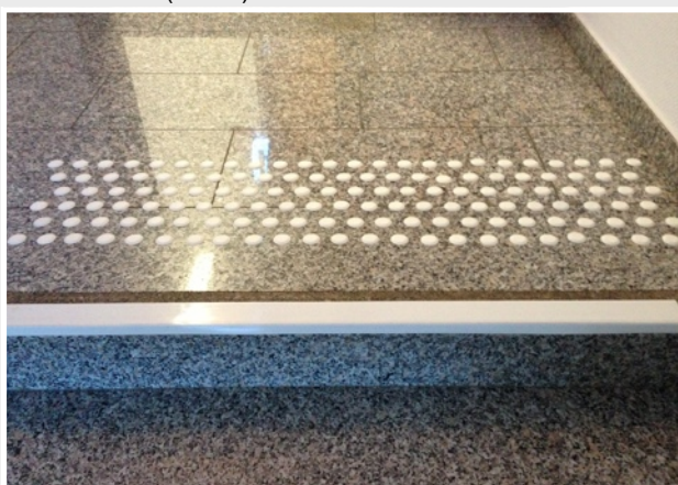
Tactile warnings consisting of domed tiles (above) or loose domes (below).
